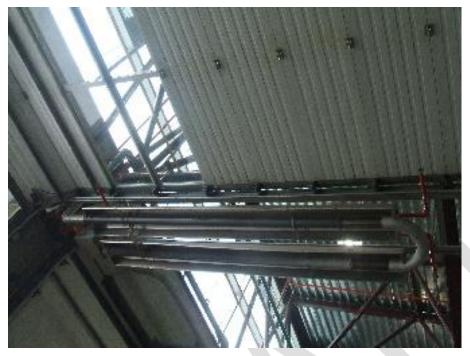
Figure 1: Infrared Heaters in the Automotive Shop
