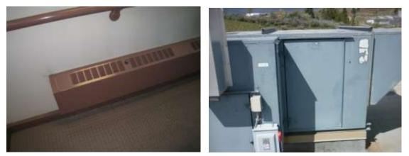
Figure 2.6 Baseboard Heater and Gas Fired RTU
