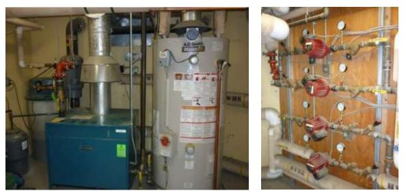
Figure 2.5 Hot Water Boiler, Domestic Hot Water Heater and Hot Water Distribution
